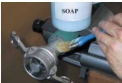
Use a lubricant to make inserting the fitting easier.
