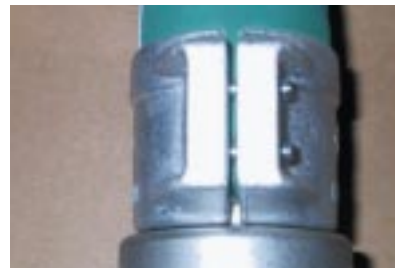
The two halves should always be parallel even when they do not get together.
